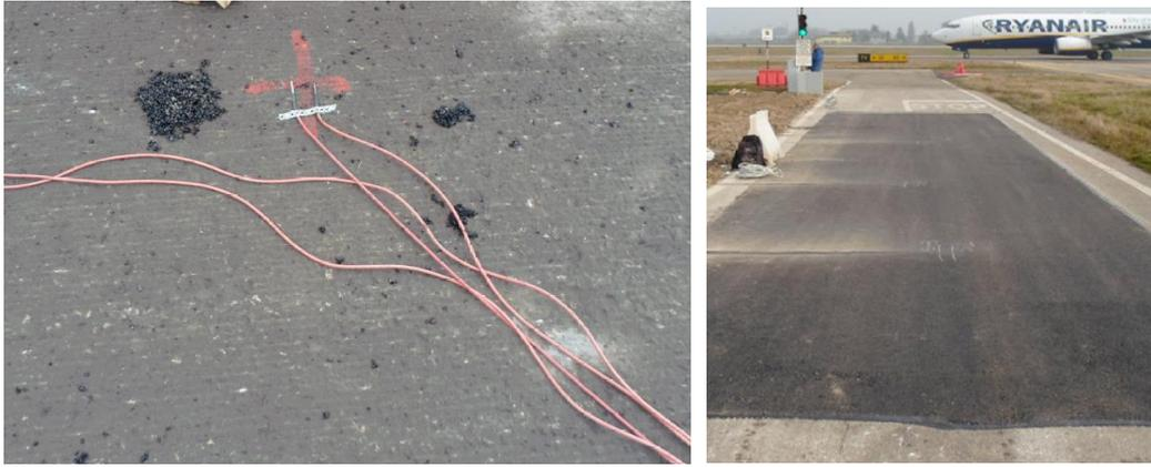
**Figure 15: Laying thermocouples on the milled surface and completed trial site**
