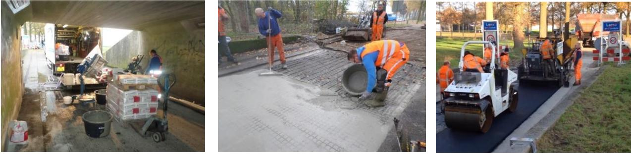
**Figure 20: Applying cement slurry and asphalt top layer**
