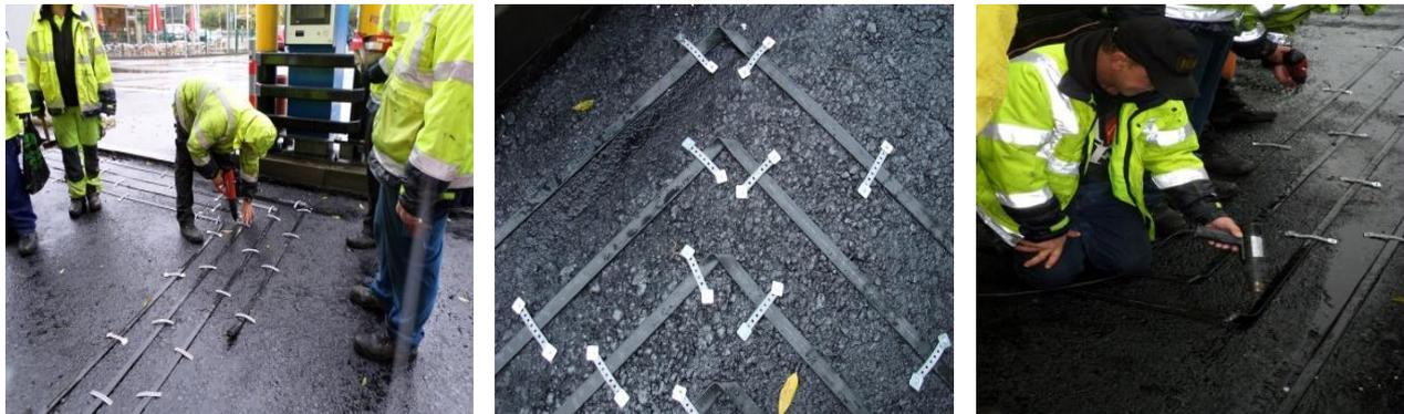
**Figure 11: Applying the infra-red ribbons to the asphalt surface with metal strips**
