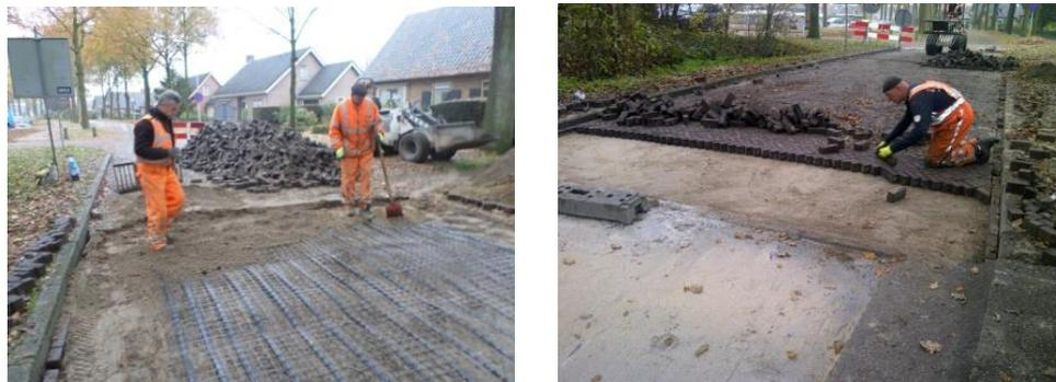
**Figure 21: Infra-red heating ribbons under block paving**
