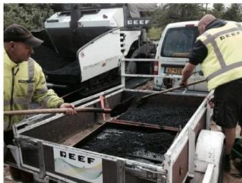
**Figure 6: Preparing asphalt slabs for laboratory measurements**
