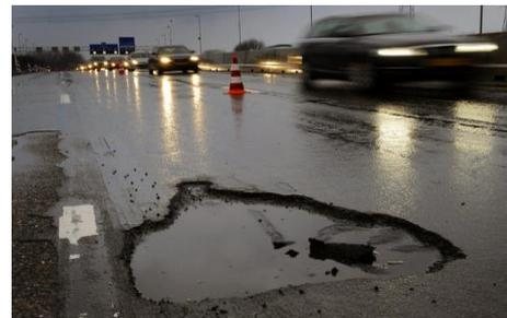
**Figure 2: Damaged asphalt surface due to winter conditions**
