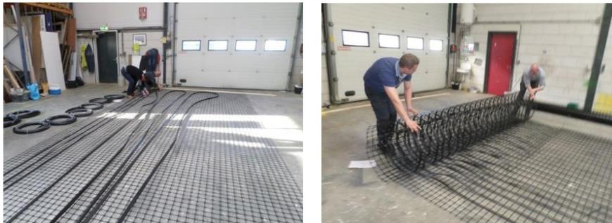
**Figure 18: Fixing the infra-red ribbons to an asphalt reinforcement mat and making it ready for transport**
