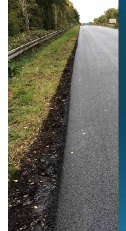
The wearing course is produced with polymer-modified bitumen, of high-quality type 40/100-75, and a high binder content. This ensures good flexibility and contributes to expected higher durability than traditional SMA wearing courses
