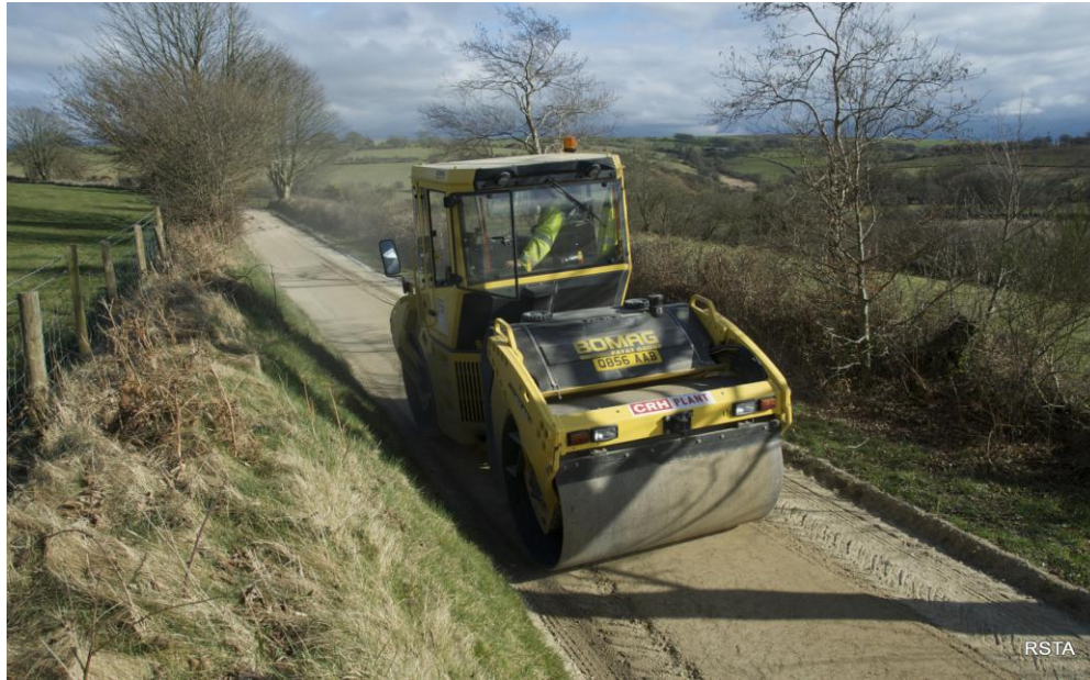
Compacting to achieve a minimum 95% of refusal density
