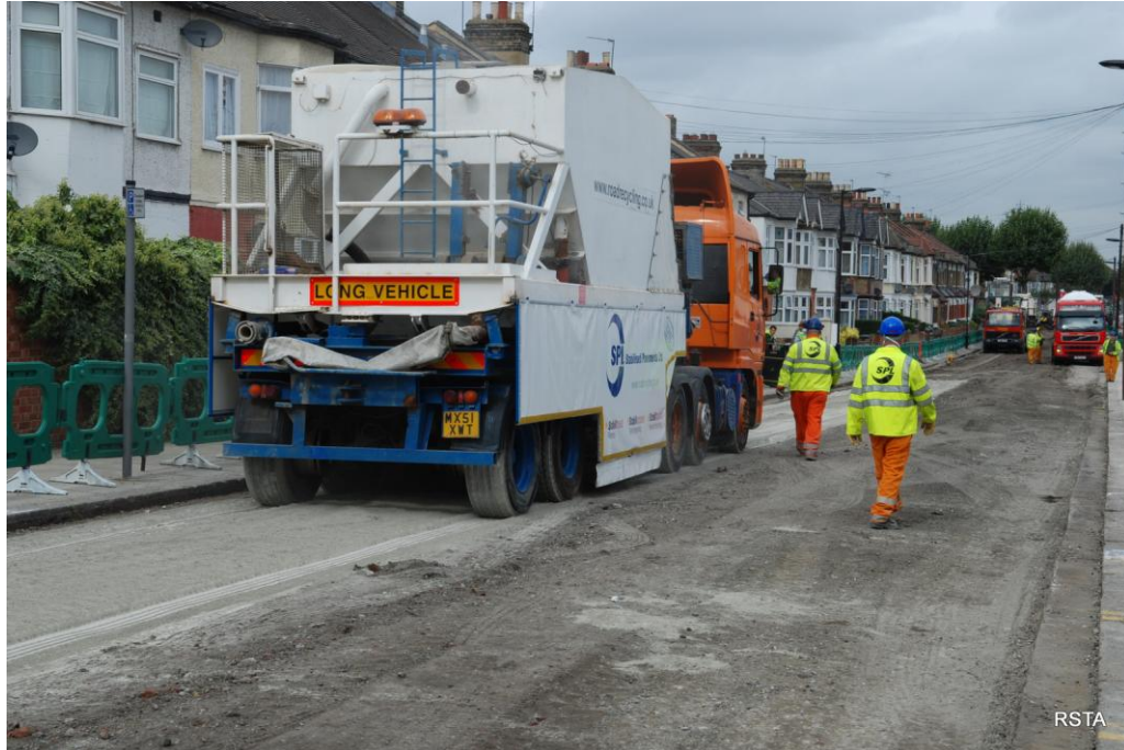
Structural Road Recycling – bulk binder spreader
