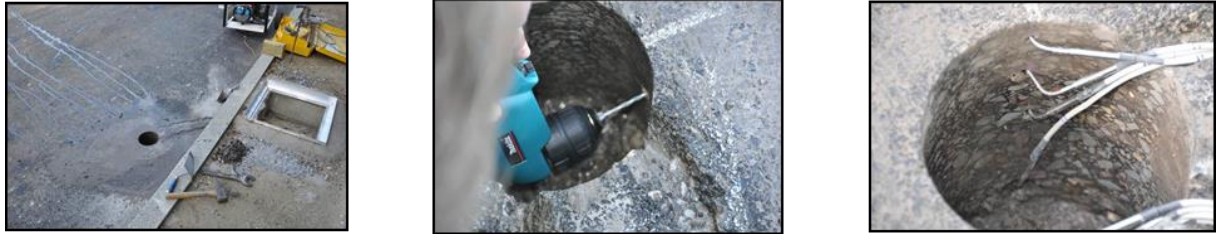
Fig 1 : Temperature sensor integration process
