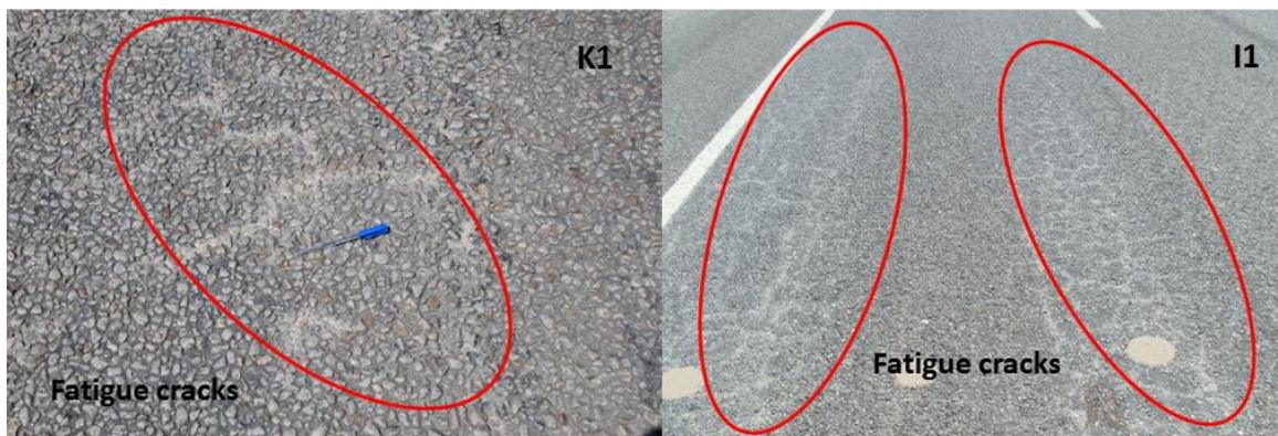
**Figure 8: Fatigue cracks at some test points**
