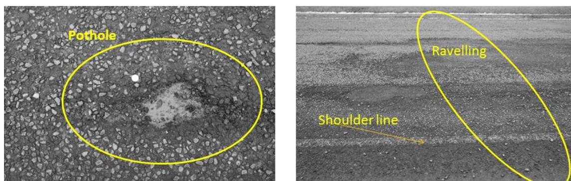
**Figure 6: Some type of deteriorations at AN1 test road**
