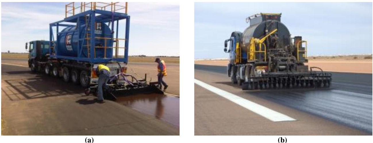
Figure 4: Surface filler applicator (a) with a squeegee and (b) without a squeegee
