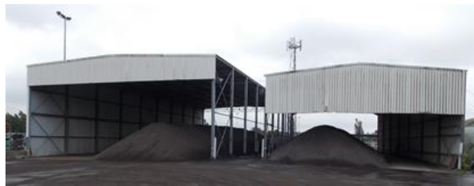
Figure 2: shed to store aggregates in order to reduce the moisture content
