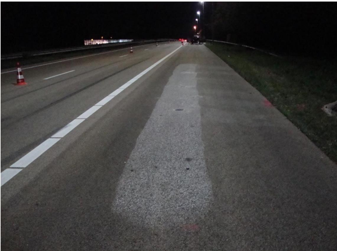
**Figure 6: Planed small section for indication of end result**
