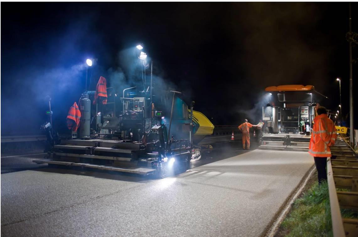
**Figure 4: Paving of light coloured asphalt**
