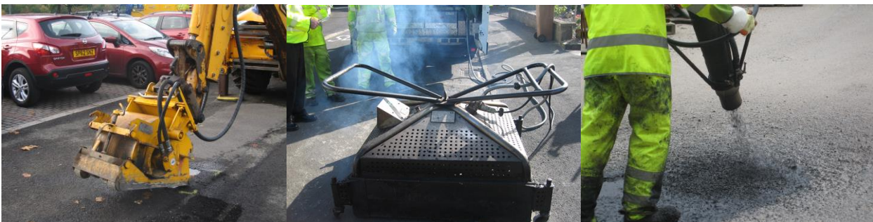
Figure 1: Examples of repair techniques: mini planer, thermal patching and jet patching.
