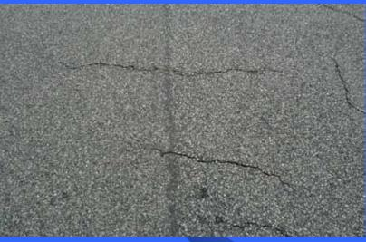
The gap-graded asphalt and the densegraded asphalt on the section with no host surface preparation, have cracked. There is no cracking what so ever in the SMA on any section. SMA is the most economical resurfacing treatment when prevention of crack propagation matters.
