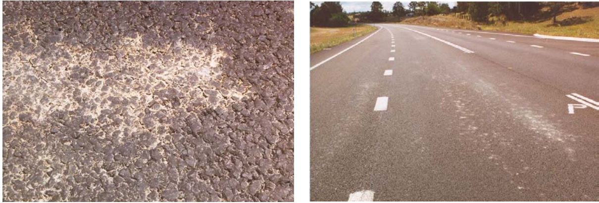
Figure 10: Asphalt deterioration due to the ingress of water in high texture surfaces with too little binder
