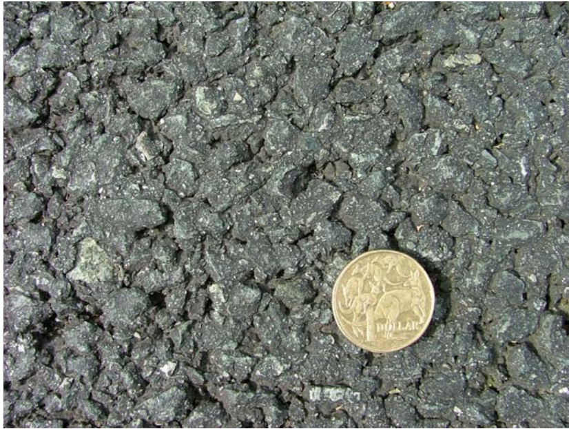
10mm GripPhalt surface texture – Kings Highway, Nelligen, NSW.
