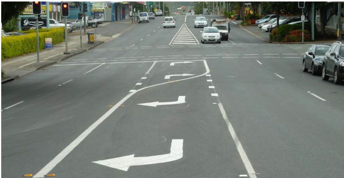
Figure 7: Photograph of DuraPave after construction
