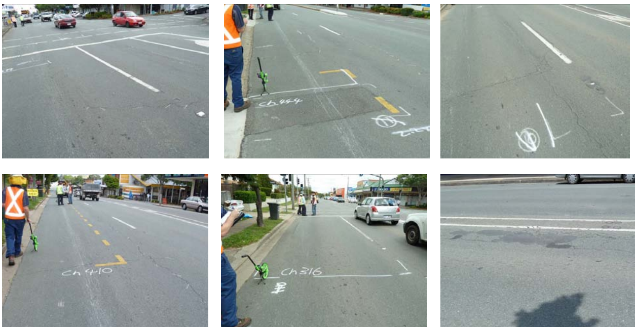
Figure 3: Photographs of existing pavement conditions
