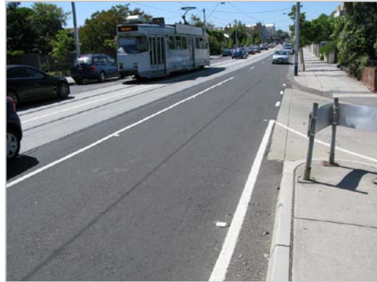
Fig. 4: Wattle tree Road in March 2010 showing no cracks
