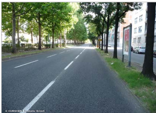
Fig. 10: HaTelit ® reinforced area in July 2009
