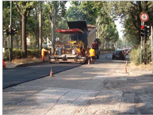
Fig. 8: Installation of 50 mm wearing course directly on concrete
