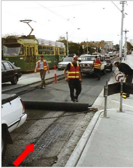
Fig. 3: Installation over construction joint due to former road widening (May 2002)
