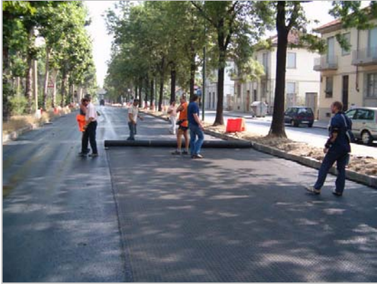
Fig. 7: Installation of asphalt reinforcement
