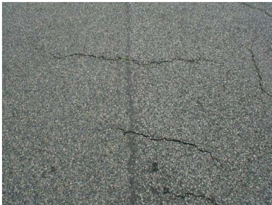
GG on right & DG on left (No host surface preparation)
