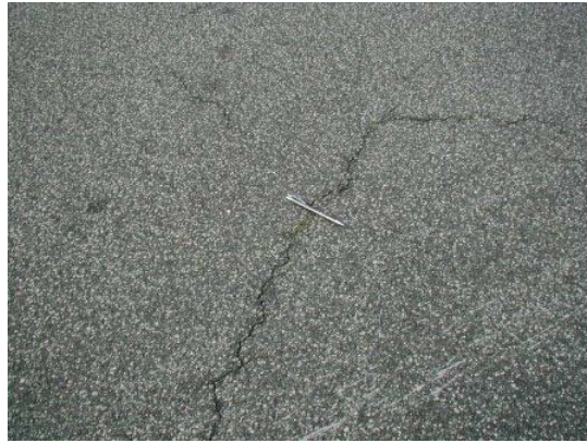
In situ recycle – No added bitumen
