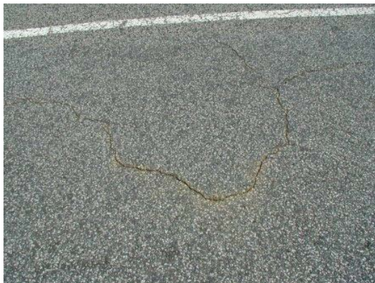
Pumping from base course (No host surface preparation)
