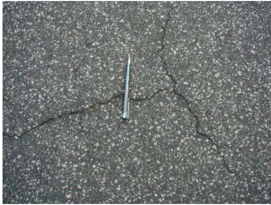
In situ recycle–2% added bitumen
