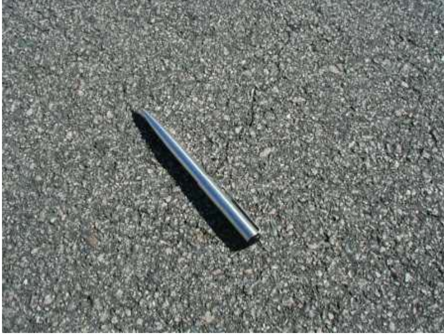
Cracking in Section 3, DG AC (after 2 years)
