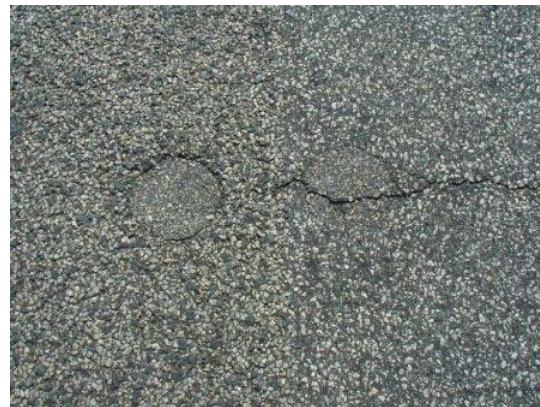
GG on right & SMA on left cored 05 (No host surface preparation)
