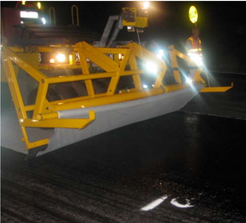
Figure 36: Laying PF1 Paving Fabric 2009
