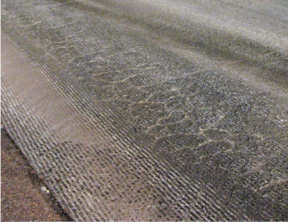
Figure 31: Existing Stabilised Pavement Base after milling
