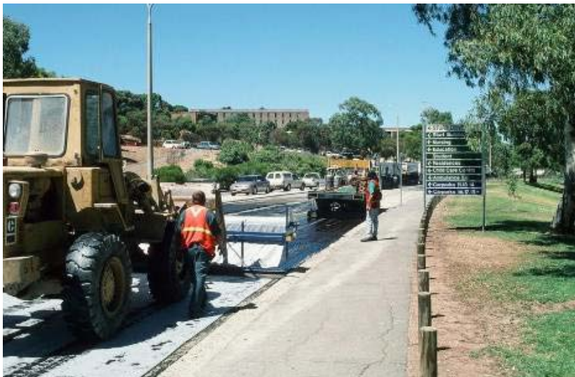
Figure 21: Laying fabric – 1999
