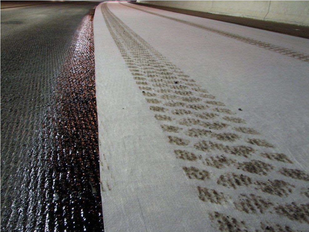
Figure 33: Paving fabric laid 2011
