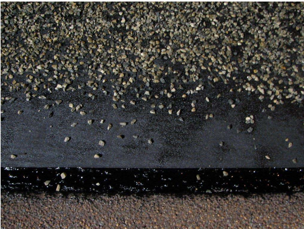
Figure 34: Paving Fabric with SAM 2011
