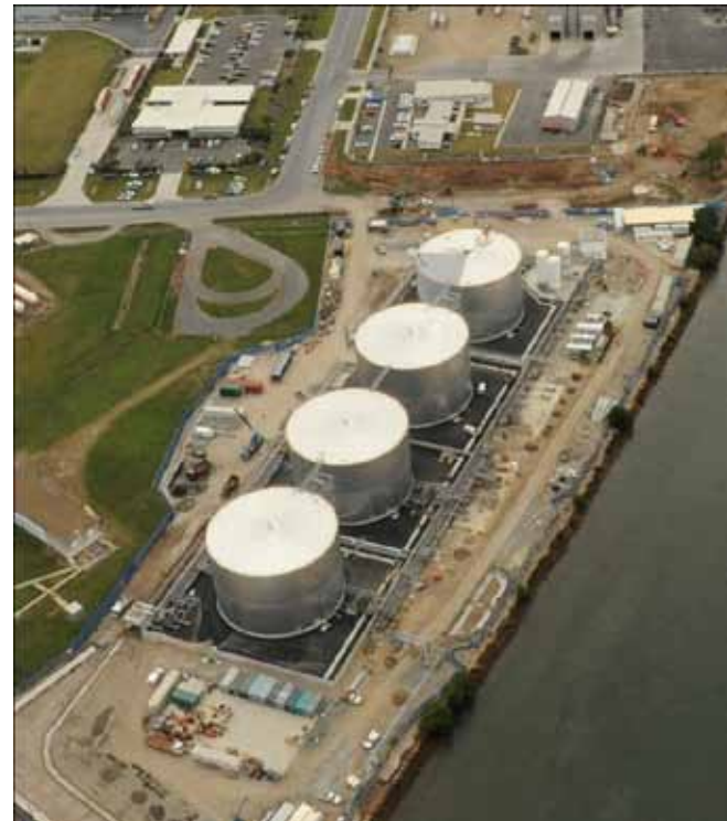
BP Storage Facility Pinkenba Qld
