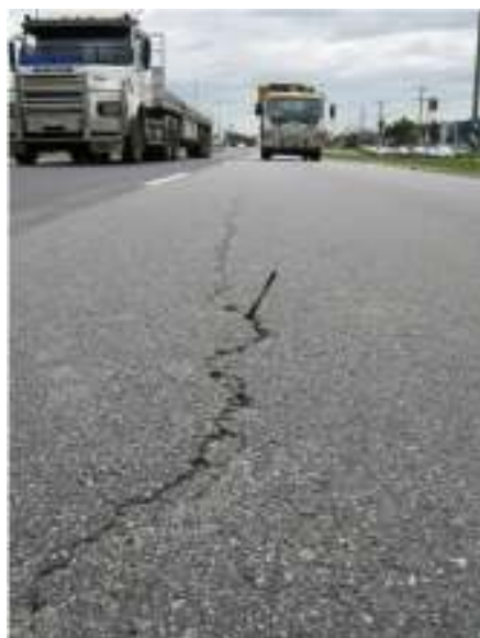
Bus bay south of intersection (Type V asphalt)
