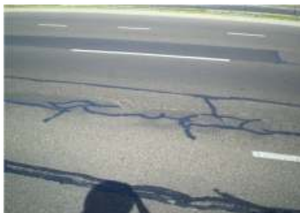
Prior to overlay
