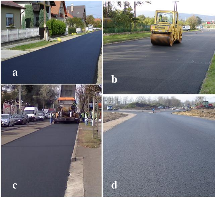
Figure 3 a-d: Asphalt wearing courses paving with AC-11 mixture containing CSRB
