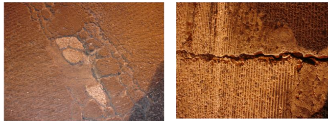
c) Longitudinal and transversal cracks.
