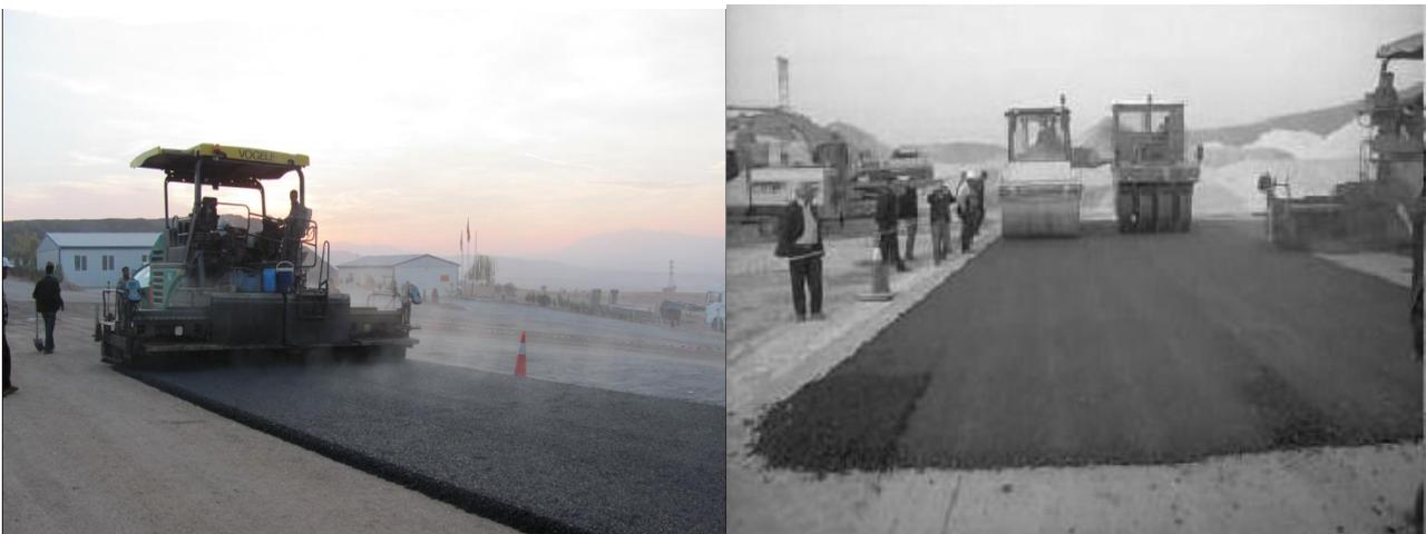
**Figure 2: The construction of binder layer**
