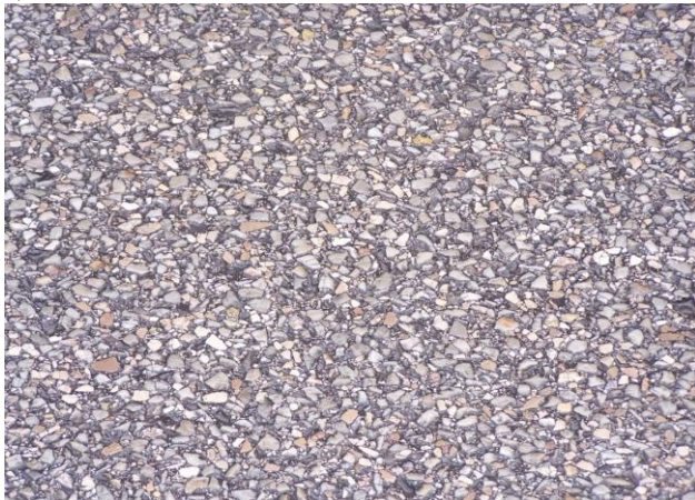
Figure 4 : View of surface texture of SMA after 12 years depending on type of adhesion agent
