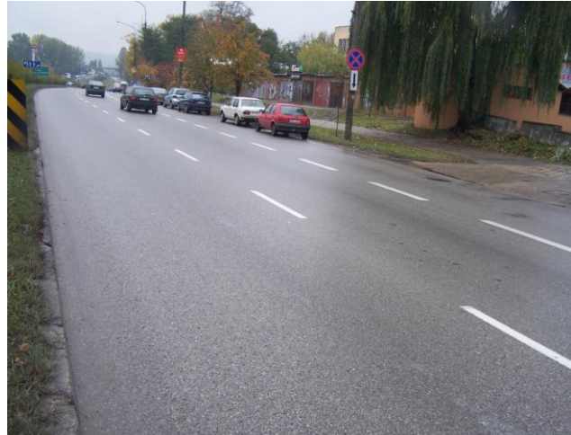
Figure 5 : View of surface of SMA after 12 years operation depending on type of adhesion agent
