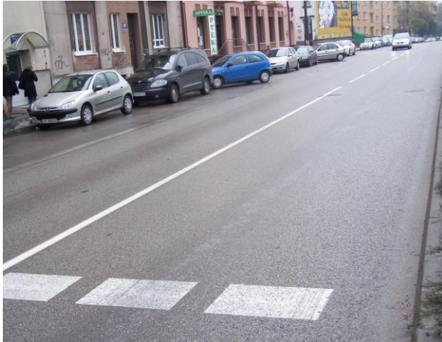
Figure 5 : View of surface of SMA after 12 years operation depending on type of adhesion agent
