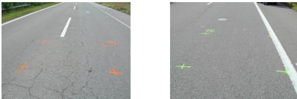
Figure 1: Road surface comparison between 2 sections after 14 years of service : highly degraded section (left) and section N°11 in good condition (right).
