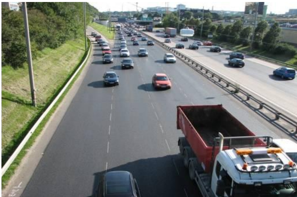
Figure 10: Asphalt Rubber (GAR 16) on a high traffic road in the Gothenburg area (E6, Ullevimotet)
