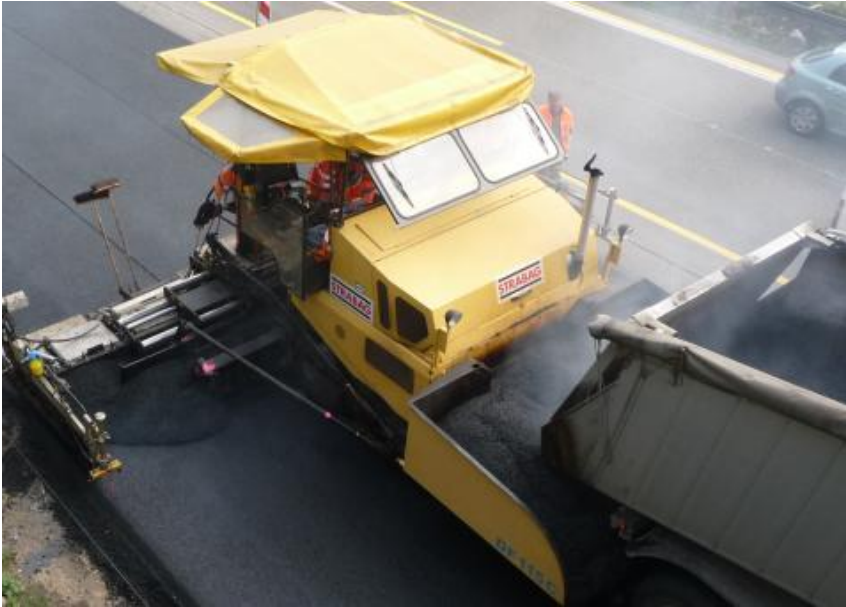
Figure 8: Paving of porous mastic asphalt
