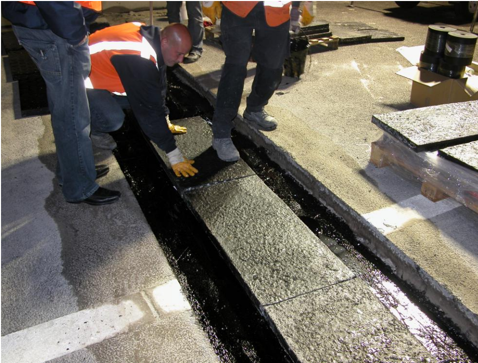
Figure 4: Second prefab element has been placed
