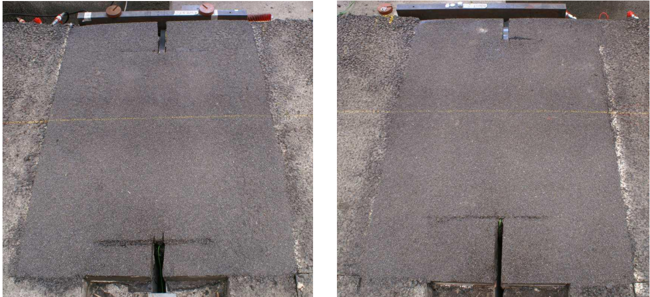
Figure 9 and 10: Joint structure after opening prior to commencing Lintrack testing (left: opening +13 mm, right: opening -13 mm)
