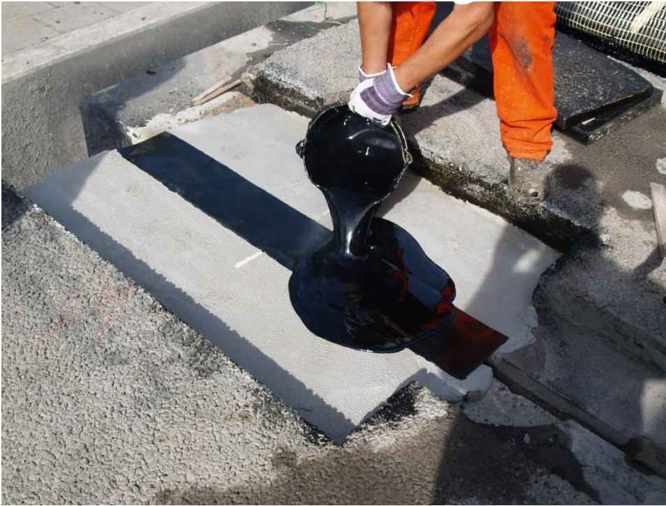
Figure 2: Pouring of hot polymer modified bitumen over the base to create adhesive layer
