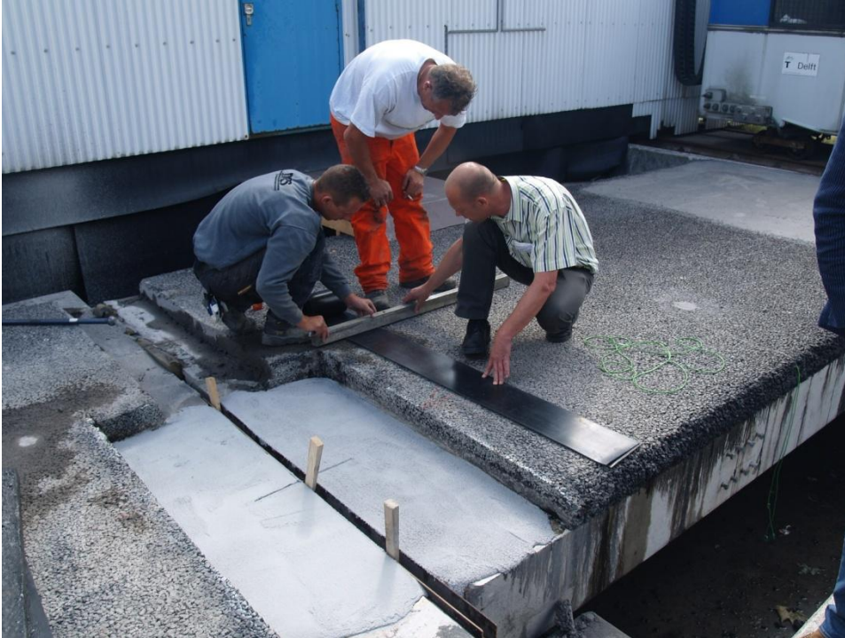
Figure 1: Preparations for covering the joint
