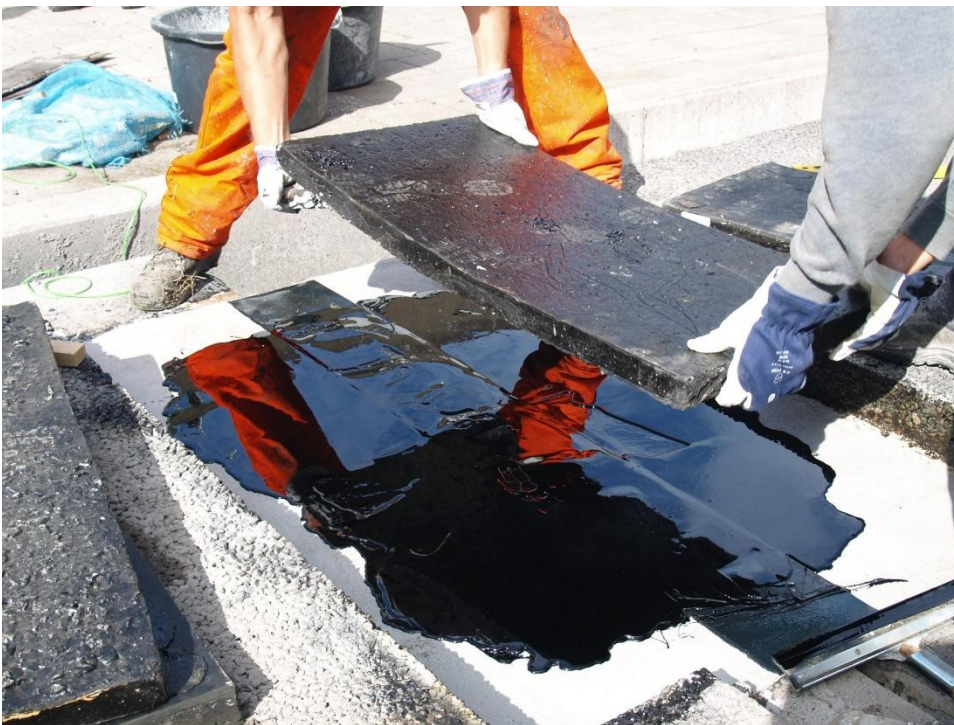
Figure 3: Placement of bottom prefab element
