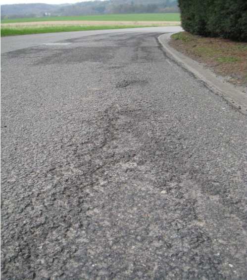
Figure 1: Material loss on an ultra-thin wearing course type UTLAC in Belgium (RUMG - Revêtement Ultra Mince Grenu)
