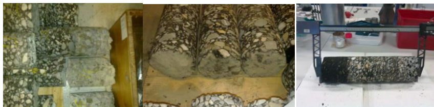
Figure 2: Left: Indication of blast furnace slag base. Centre: Indication of sand sub-base. Right: measurement of total asphalt thickness.
