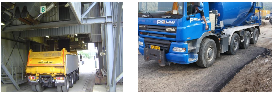
Figure 9 : Asphalt plant – truck loading [left], heavy transport on freshly laid Greenway LE asphalt [right]
