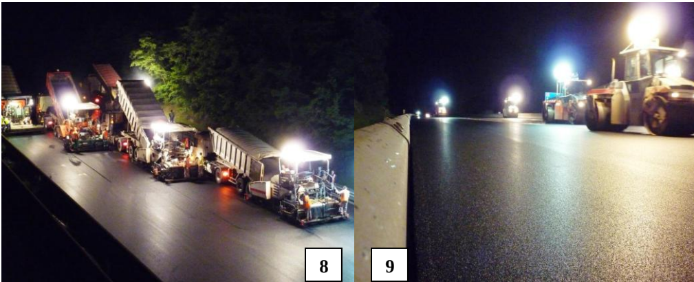
Figure 8: Laying of equipment.
