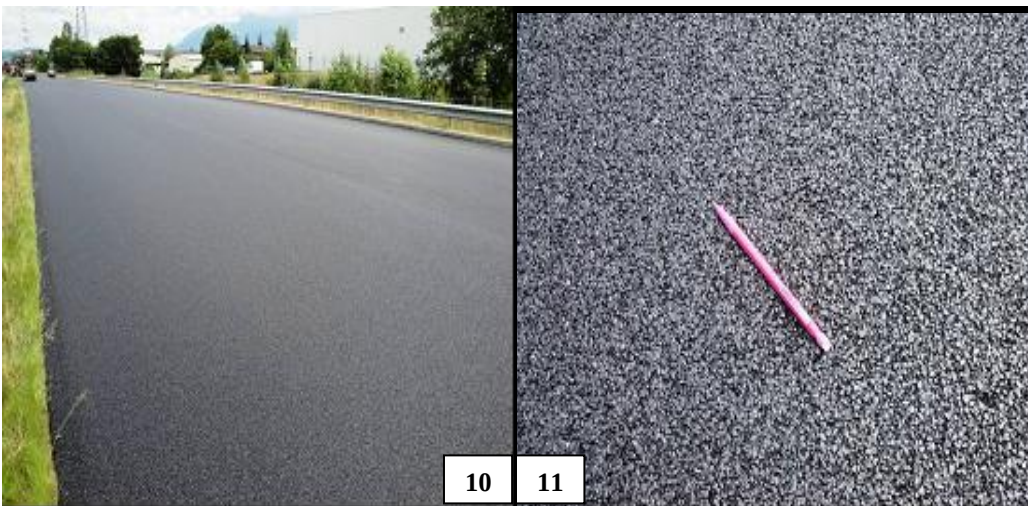
Figure 10: Overview of the worksite
