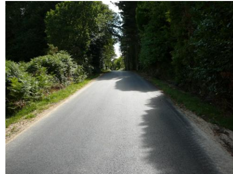
Picture 5 : Re-profiling works
