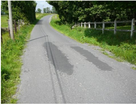
Picture 4 : Repair of potholes
