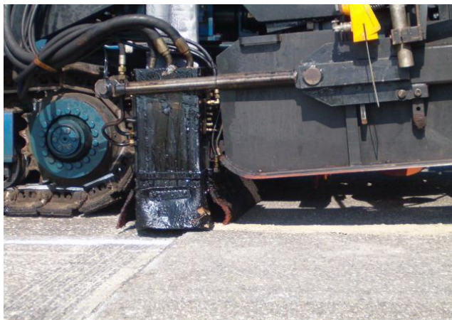
Photo 3: Paver with integrated spray bar.
