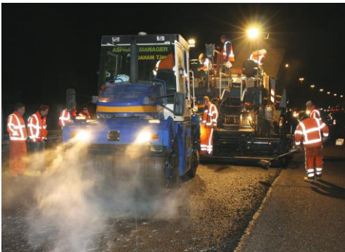
Photo 6: Overview of the laying process.
