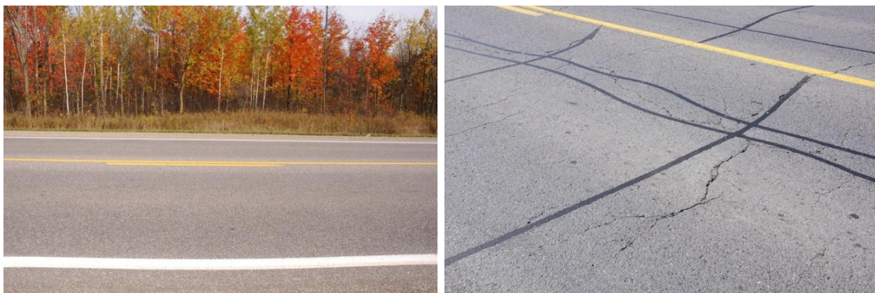
FIGURE 1 – Performance variation for bitumens of nearly identical Superpave grades but different rheological type (sol-type versus gel-type). Note: These are representative photographs for adjacent paving contracts. The first was constructed in 2000 with polymer-modified bitumen whereas the second was constructed in 1998 with bitumen blended with WEO residue. The poor performer carries only about 60% of the average daily traffic compared to the good performer. The only explanation for this huge performance difference was found to be the difference in bitumen rheological type and thus quality [17].
