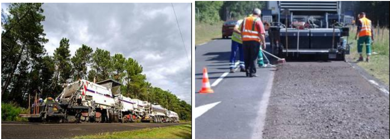
Figure 2 – Recycling work in progress
