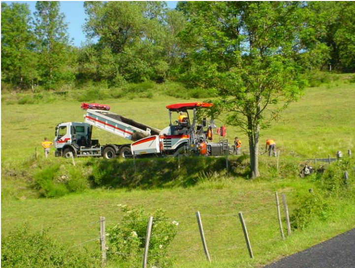
Figure 3. Laying the 100 % RAP-based asphalt mix on the jobsite in the Auvergne region
