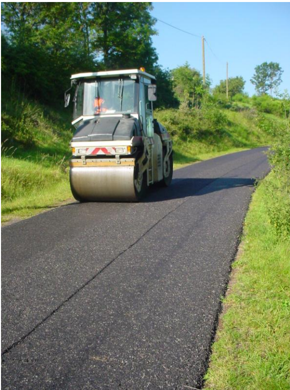
Figure 4. Compaction of the 100 % RAP-based asphalt mix on the jobsite in the Auvergne region
