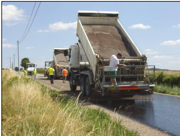
Figure 1: Low granularity surface dressing laying – RD5
