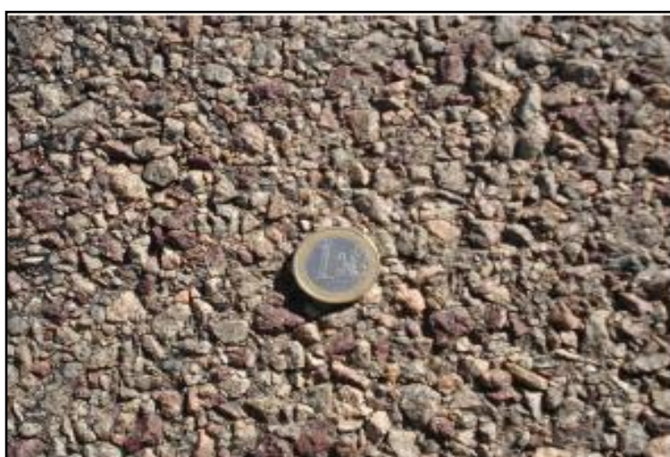
Figure 4 : Visual appearance of a single 4/6-2/4 mm (double chipping) surface dressing.
