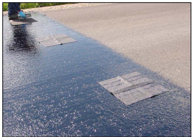
Figure 3 : Bitumen proportioning control
