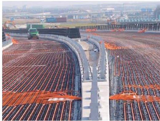
Figure 2 – Asphalt collector in Rotterdam [3].
