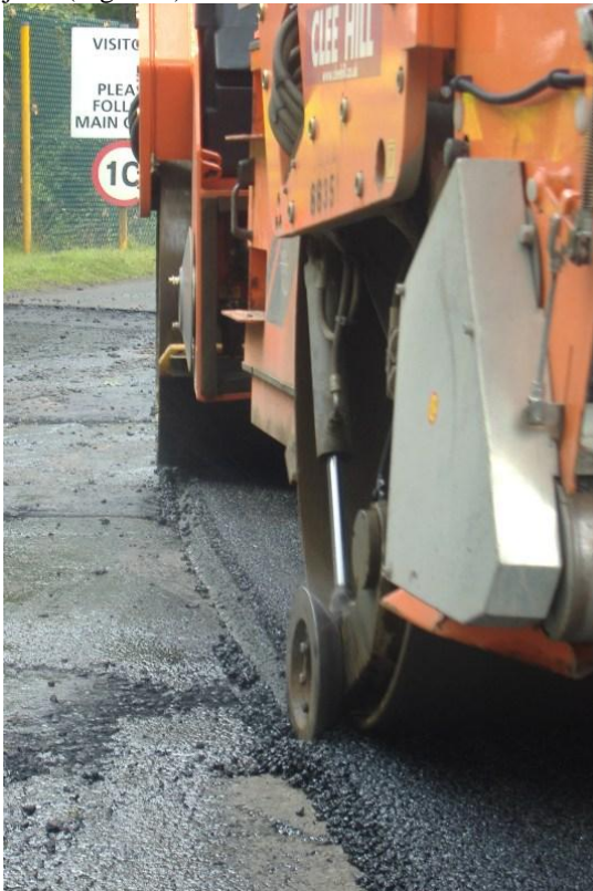
Figure 4: Chamfered Joint with roller in 'Crab-steer'
