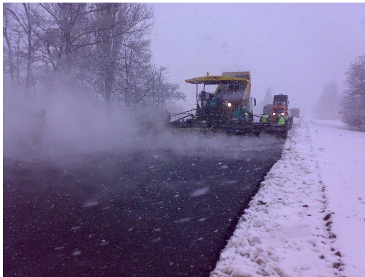
Figure 3. Asphalt layers paving in below 0°C conditions
