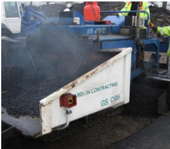
Figure 9: Material being laid through a minipaver
