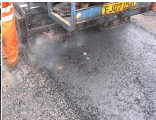
Figure 10: Material containing 11% UVO, laid through a minipaver
