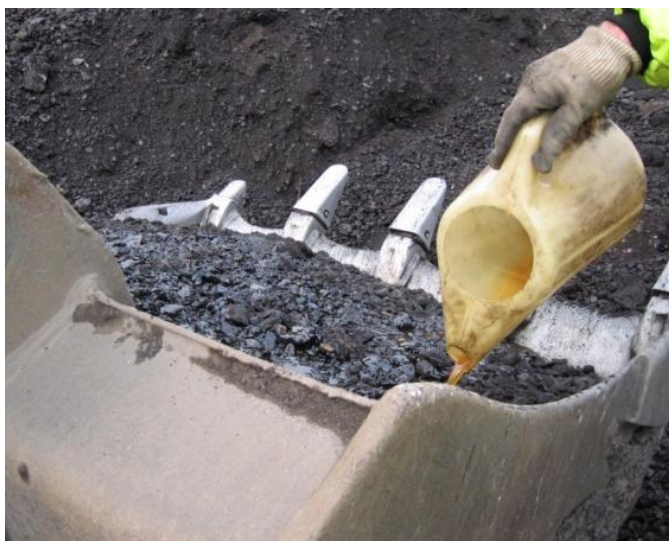
Figure 7: UVO added to the bucket of the loading shovel prior to mixing
