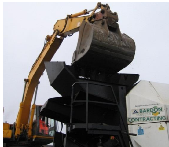
Figure 6: Loading material into the recycler
