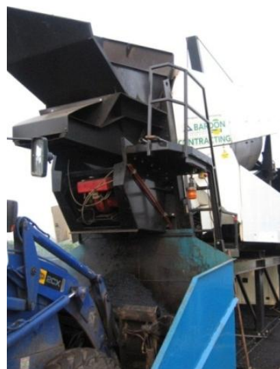
Figure 8: Emptying of the material from the hot mix recycler
