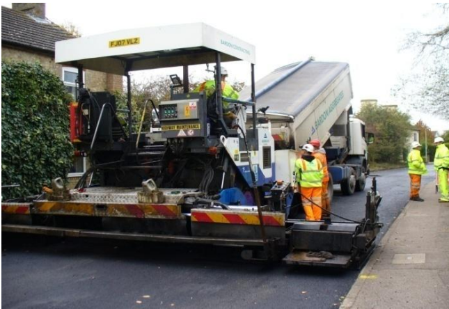
Figure 5: Laying of AC10 close surf 70/100 Control
