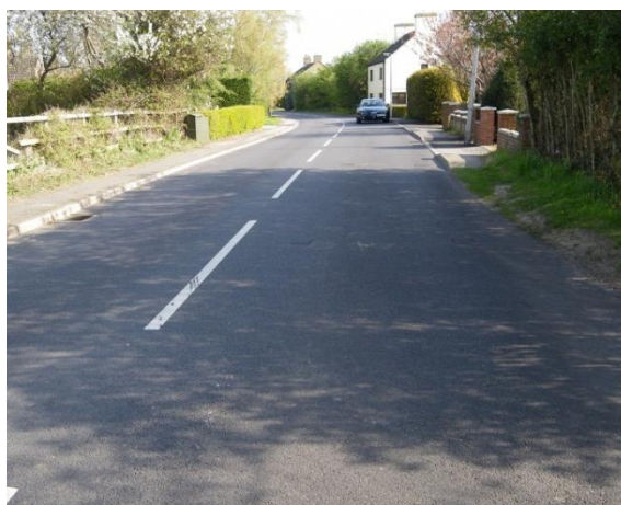
Figure 10: Vegetex material, New Road approach to the village.
