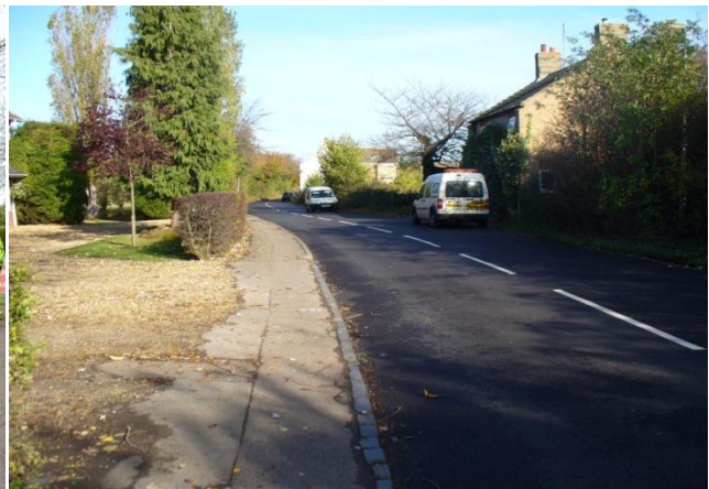
Figure 6: Compacted AC10 close surf 70/100 Control
