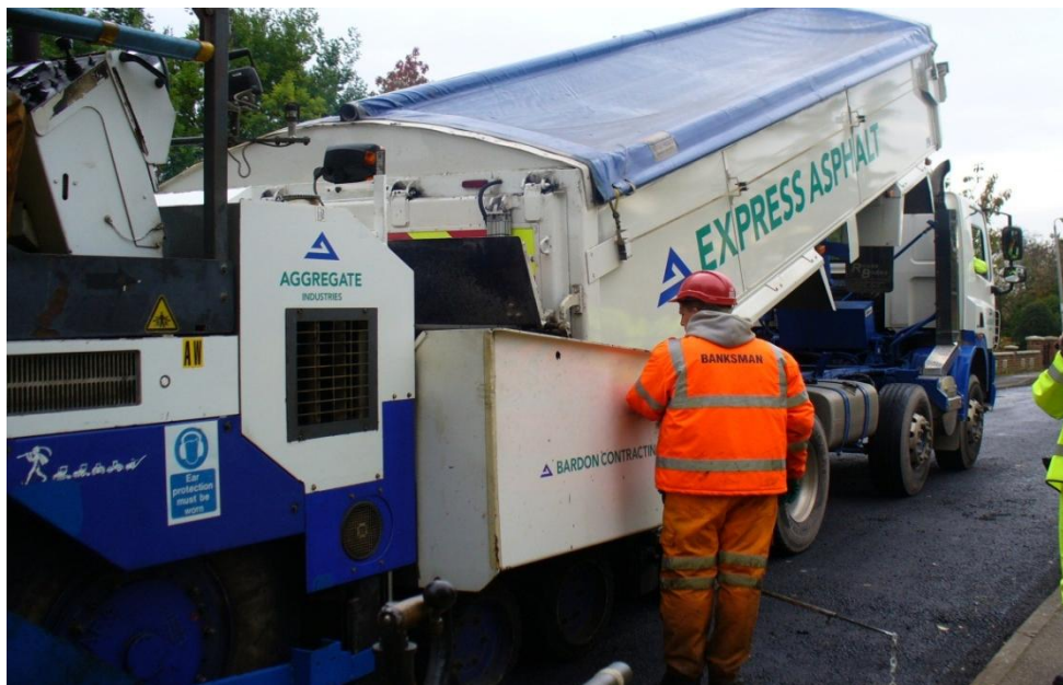
Figure 7: Laying of AC10 close surf Vegetex 85
