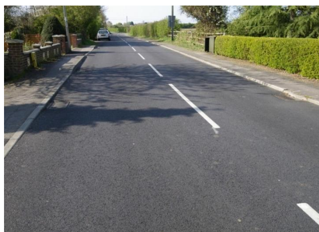
Figure 11: Vegetex material, New Road leaving the village.
