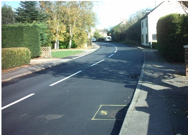
Figure 8: Compacted AC10 close surf Vegetex 85
