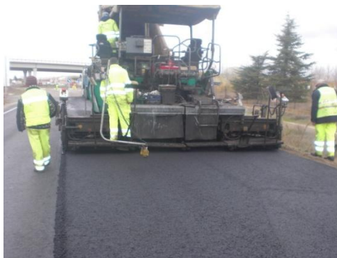
Figure 3. Paving without fumes
