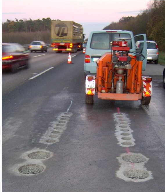
Figure 1: Core excavation from a highway section
