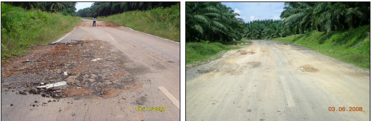
Figure 8 - Pavement defects
