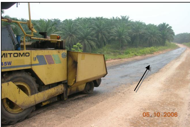
Figure 5 - Prime coating
