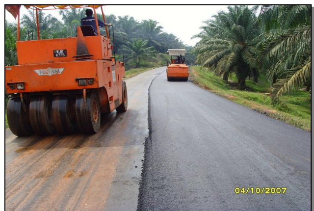
Figure 6 - Compaction of ACWC
