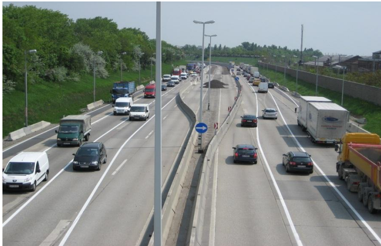
Figure 4: Narrowed lanes, northbound and southbound carriageway (Photo ASFiNAG)
