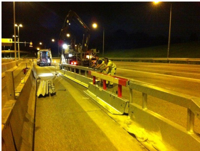
Figure 7: Installation of emergency doors (Photo ASFiNAG)
