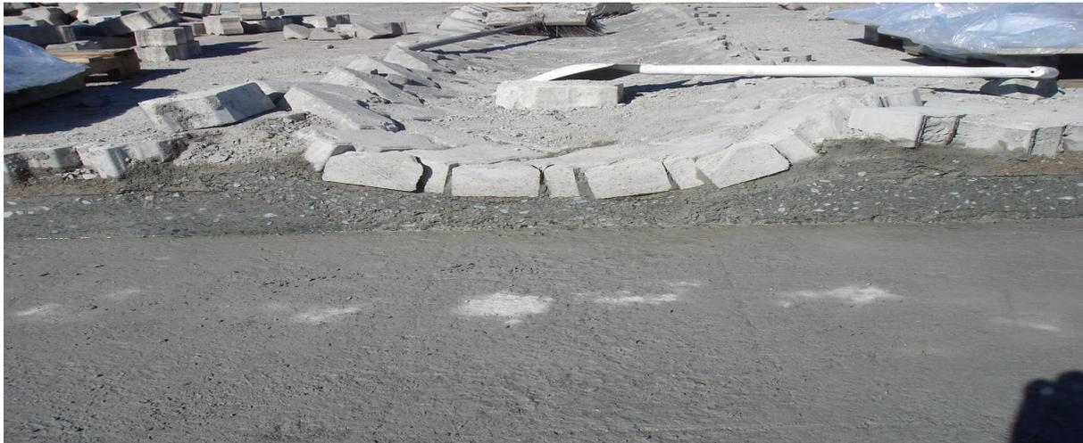
Photo 2 Rutting Limited to Base Layer
