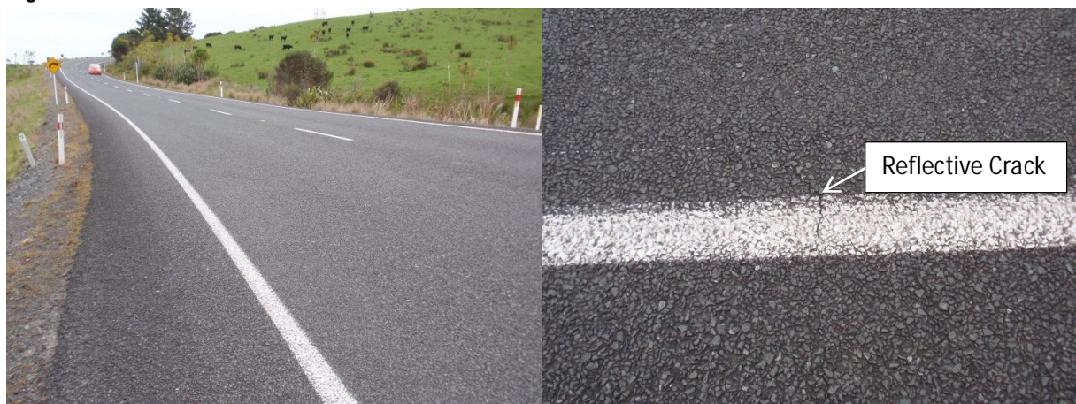
Figure 17 – Surface of Cement Bound Basecourse at Nine Years' Service
