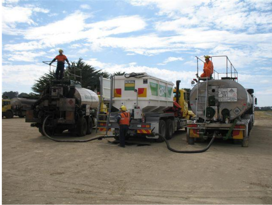
Figure 2 Field blending of conventional crumb rubber bitumen
