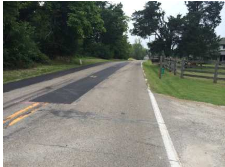
Condition before paving
