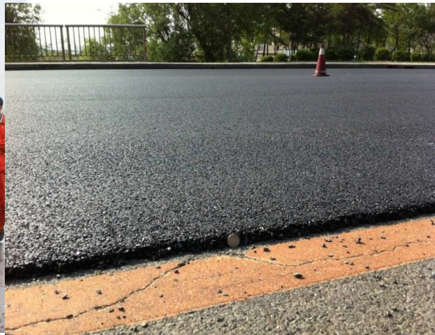
2.5 cm thick after compaction
